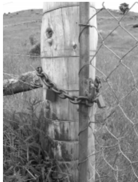
The locked gate, lacking any signage. When a gate is erected across a public road, Section 344(2) of the Local Government Act 1974 requires the person authorised to erect the gate, or at whose cost it has been agreed that the gate shall be erected and maintained, to fix a board upon each side of the gate, with the words 'Public Road' legibly painted in letters of not less than 75 millimetres in height.
